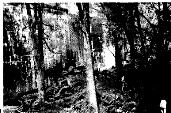
FIG. 2. Moore Creek Dam (1898): (a) Cross Section of Dam Arch; (b) View from Right Bank of Downstream Vertical Wall (1997 Photograph); (c) View from Downstream Showing Overfall Spillway Section, with Scour at Bottom of Wall behind Leftmost Tree (1997 Photograph)
