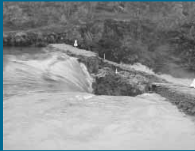
Breaching a 6m high embankment in Norway (Oct. 2002)
