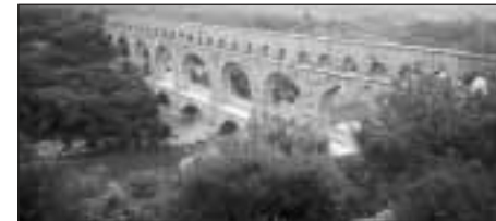
Fig. 1 - Pont du Gard, Nîmes aqueduct in June 1998 - Looking from the right bank
