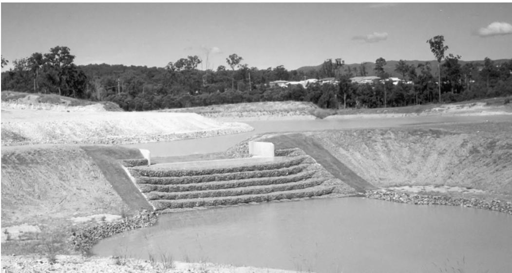
Figure 7. Gabion stepped spillway at Robina (Gold Coast QLD, Australia) on 2 April 1997, shortly after completion:  $h \sim 0.5$  m,  $h/l \sim 0.5$
