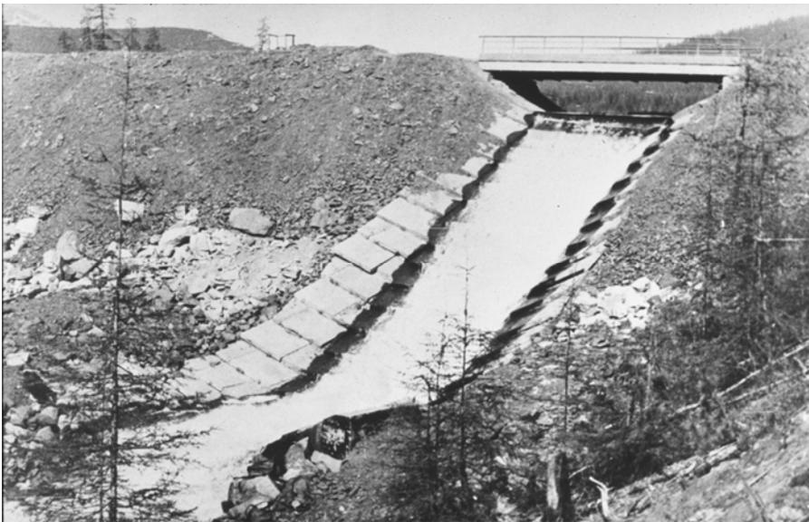
Figure 8. Precast concrete block spillway of Volymia dam (Siberia, Russia) (Courtesy of Prof. Y. Pravdivets) - This experimental structure (H=20 m) operated for more than 15 years, the spillway discharging ice and water from early spring to late fall
