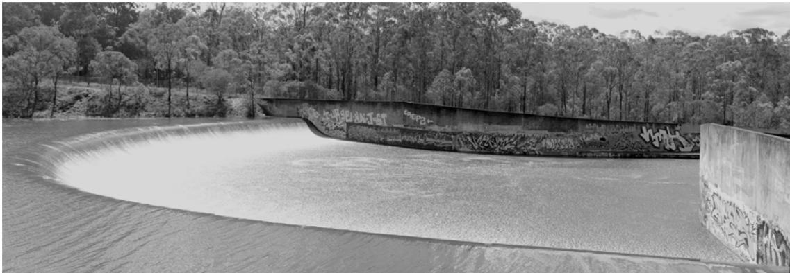
Figure 4. Minimum energy loss spillway inlet at Lake Kurwongbah (Brisbane QLD, Australia) in operation on 29 January 2013
