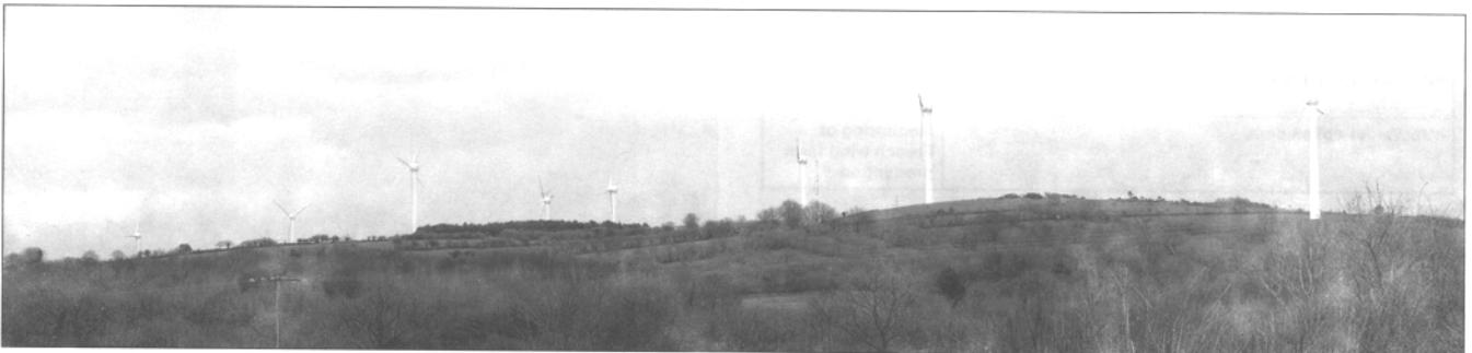
Figure 7. Wind farm at Plougras, Monts d'Arrée, Côtes d'Armor on 27 February 2004, during a Northerly breeze. Installation was completed in 2003, with 8 turbines and a total capacity of 6 MW. Noise problems were experienced at the start in June 2003, but were fixed in October 2003 after a lot of "bad press."
