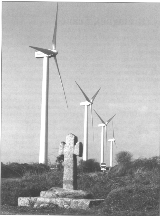
Figure 3. Wind farm at Plouarzel, Pays du Léon. Photo shows turbines on 1 March 2004 with only 4 rotors out of 5 operating during a moderate, easterly breeze. Each mast is 38.4 m high and weights 28.9 tons. Installation was completed in 2000, and has 5 turbines with total capacity of 3.3 MW. Production is 9,800 MWh per year.
