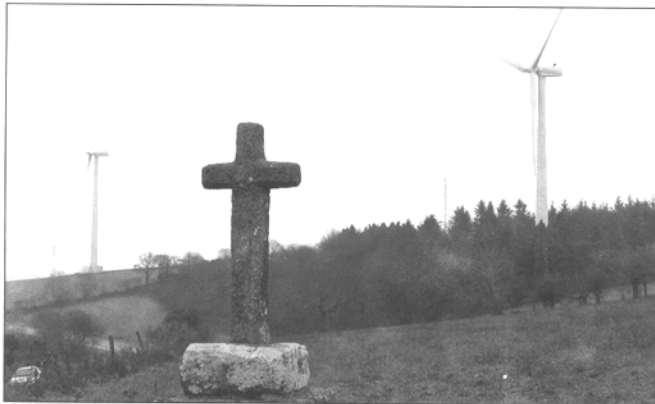
Figure 3. Wind farm at Plouarzel, Pays du Léon. Photo shows turbines on 1 March 2004 with only 4 rotors out of 5 operating during a moderate, easterly breeze. Each mast is 38.4 m high and weights 28.9 tons. Installation was completed in 2000, and has 5 turbines with total capacity of 3.3 MW. Production is 9,800 MWh per year.
