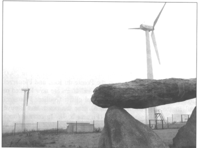
Figure 5. Privately-owned and operated wind farm at Beuzec-Cap-Sizun, Cornouaille. Installation was completed in 2001, and has 5 turbines with total capacity of 1.5 MW. Noise problems were experienced and the station was shut down. Photograph taken on 3 March 2004, when all rotors were stopped. Note that the turbines are closely located to each other and interactions between rotors could be expected.
