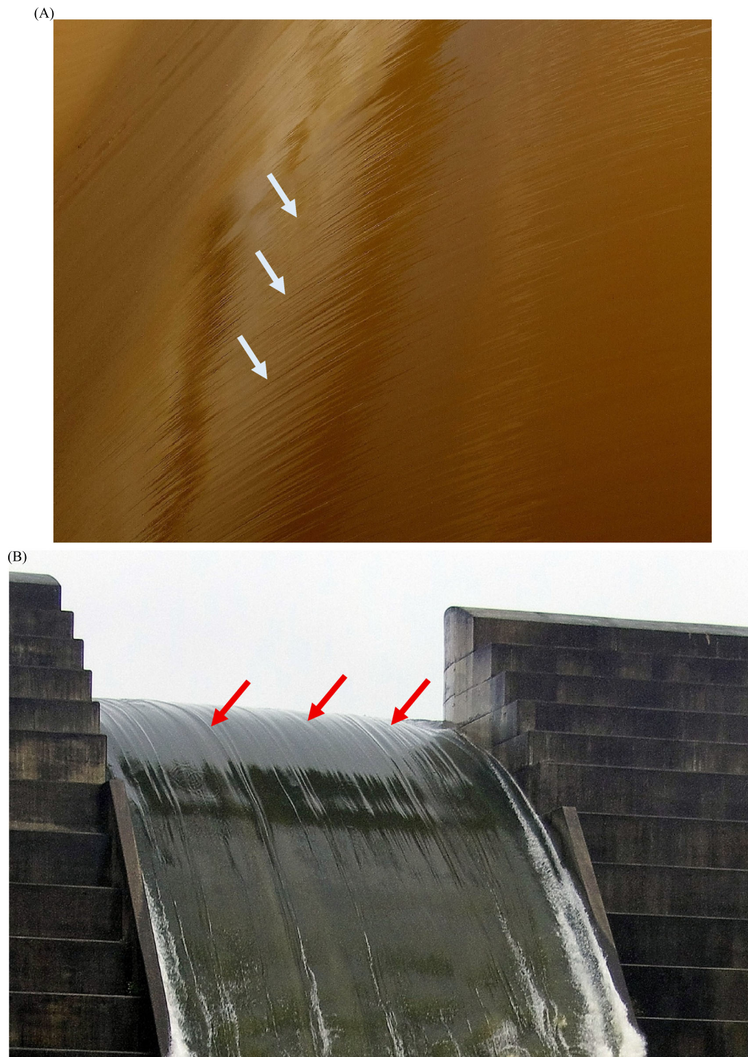
Figure 2. Longitudinal free-surface striations and surface scars in prototype chute spillways with uncontrolled crest during large flood events (Photographs Hubert Chanson). (A) Surface striations (light blue arrows) immediately downstream of the crest at Burdekin Falls Dam spillway (North Queensland, Australia) – Q = 13,700 \text{ m}^3 \text{ s}^{-1} , Re = 1.1 \times 10^8 , shutter speed: 1/8000 \text{ s} , aperture f2.4, 13 February 2025 – flow direction from right to bottom left. (B) Surface striations (red arrows) at Hinze Dam spillway (south-east Queensland, Australia) – Q = 116 \text{ m}^3 \text{ s}^{-1} , Re = 4.2 \times 10^7 , shutter speed: 1/200 \text{ s} , aperture f5.6, 27 February 2022 – flow direction from top left to bottom right.
