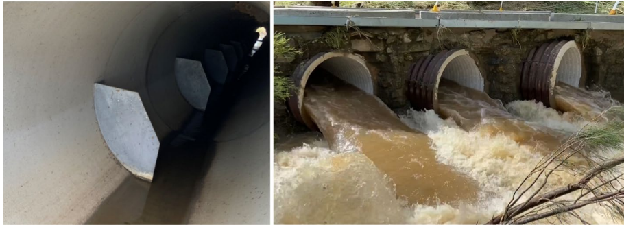
Fig. 1 Smooth circular pipe culverts located on fish-mapped waterways [8]. (LEFT) “Quad” baffles fitted to a 1050 mm diameter reinforced concrete pipe culvert at Walloon, Queensland, Australia (RIGHT) Outlet flow from a 3/1500 mm diameter slip-lined pipe culvert at Brookfield, Queensland, Australia after a storm event on 28th February 2022
