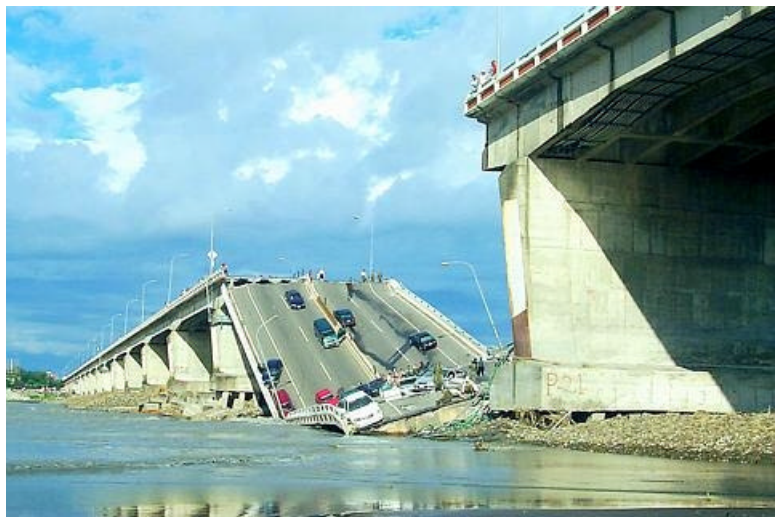
Fig. 2-1 - Bridge failure between Kaohsiung and PingTung city on the Kaoping river (Taiwan, 27 Sept 2000) (Courtesy of HUANG L.C., The Liberty Times)
