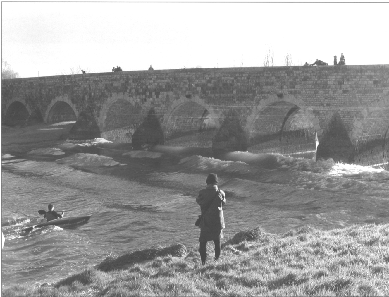
Figure 7. Photograph of the Sélune River tidal bore on 7 April 2004 at Pontaubault (low tide: 0.90 m, high tide: 14.55 m). Looking at the advancing tidal bore (mascaret) passing below the 15th century Pont Aubaud. Note the bridge piers are shaped to cut the bore front.
